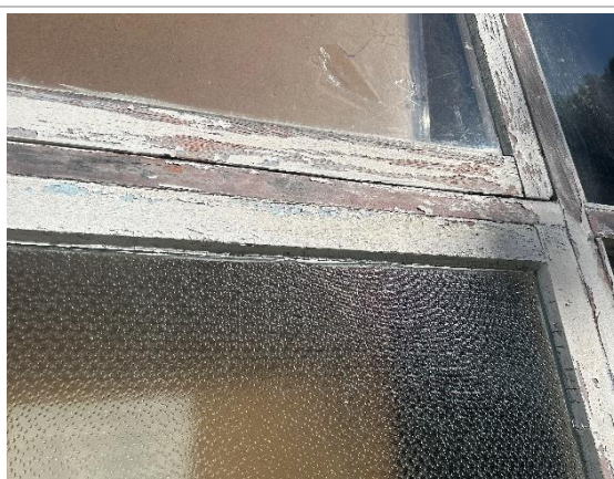
Photograph 3: Paint flaking on joinery indicating possible lead based primer.
