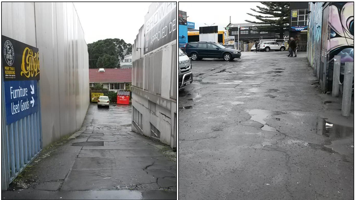
Photographs 2 and 3: Areas of cracked and patched asphalt at the 216 Dominion Road accessway (left) and the 117 Valley Road accessway (right).
